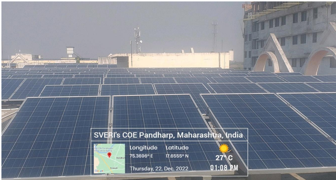
400 kw Solar Roof top Plant
